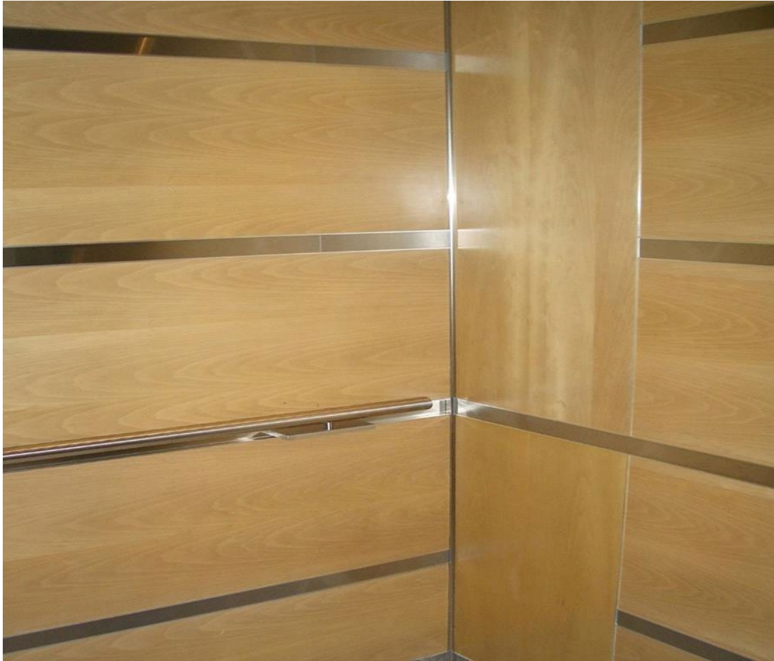
Golden Sassafras veneer on Flameblock in a lift car interior - Group 2
